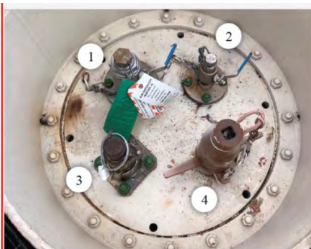
Top Connections & Valves
